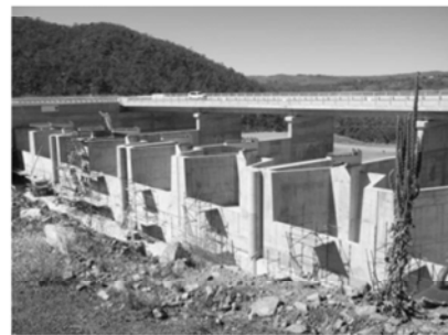
Fig. 7 Auxiliary spillway from upstream
