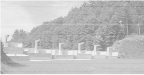
Fig. 12 Otter Brook fusegates from upstream
