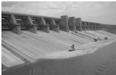
Fig. 9 Service spillway from downstream
