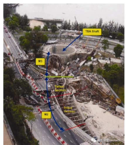
图 13 Nicoll highway 基坑倒塌现场 [4] Fig. 13 Nicoll highway excavation after collapse [4]
