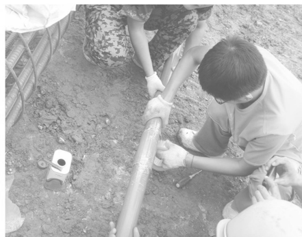
(c) 测斜管安装
